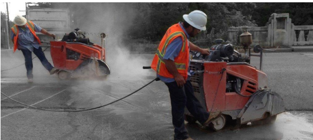
“Dusting” caused by operators reducing water feed to the blade when using Road Saws currently on the market in an effort to reduce slurry clean-up.
