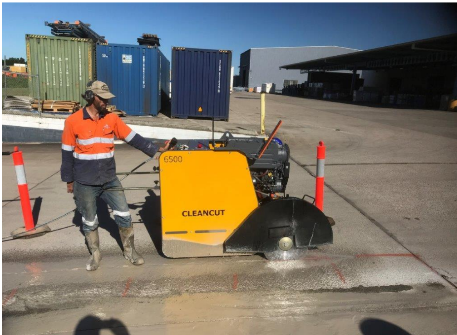
The Cleancut Slurry Recycling System and Flowmeter solves the “Dusting Issue.”
